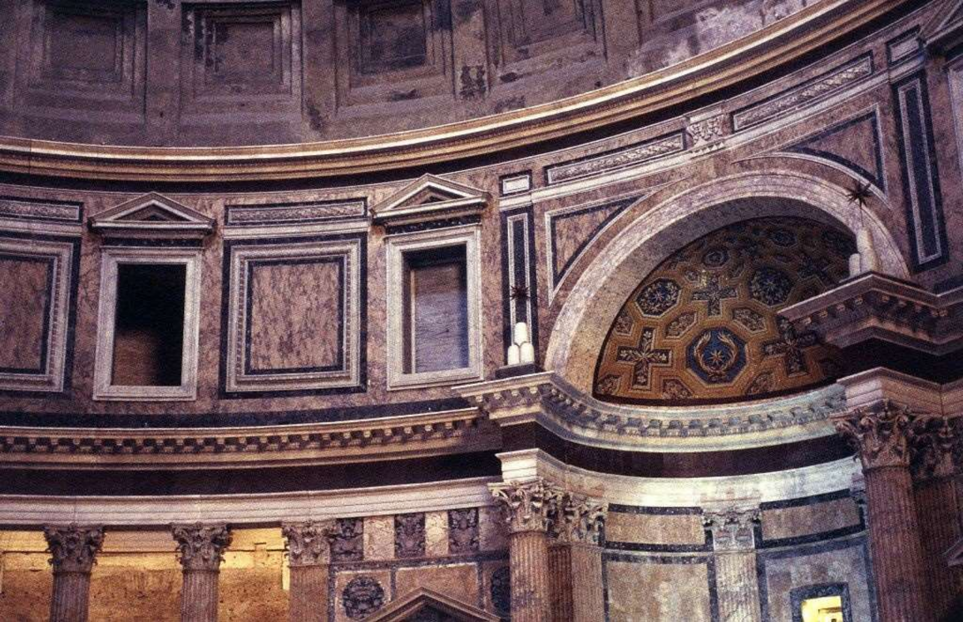
Interior detail: Wall decoration with pediments over niches
