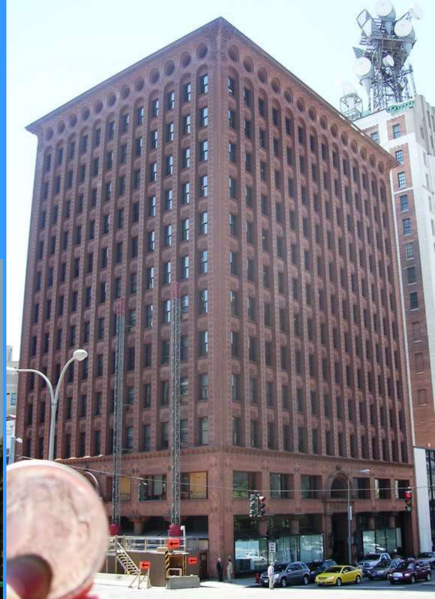
Louis Sullivan, Guaranty (Prudential) Building , Buffalo, NY, 1894-1896.
