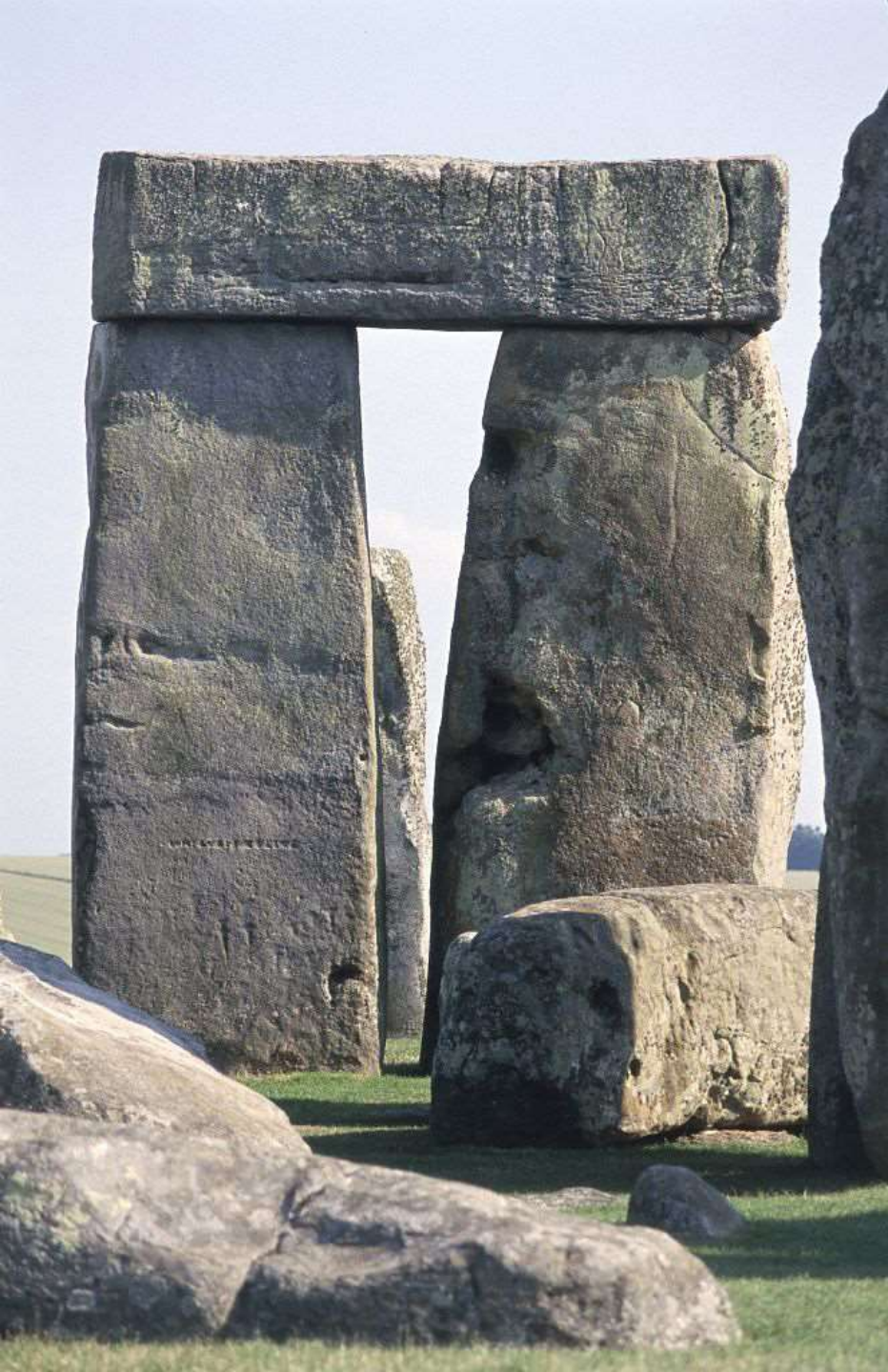
1.24 Post-and-lintel construction.
