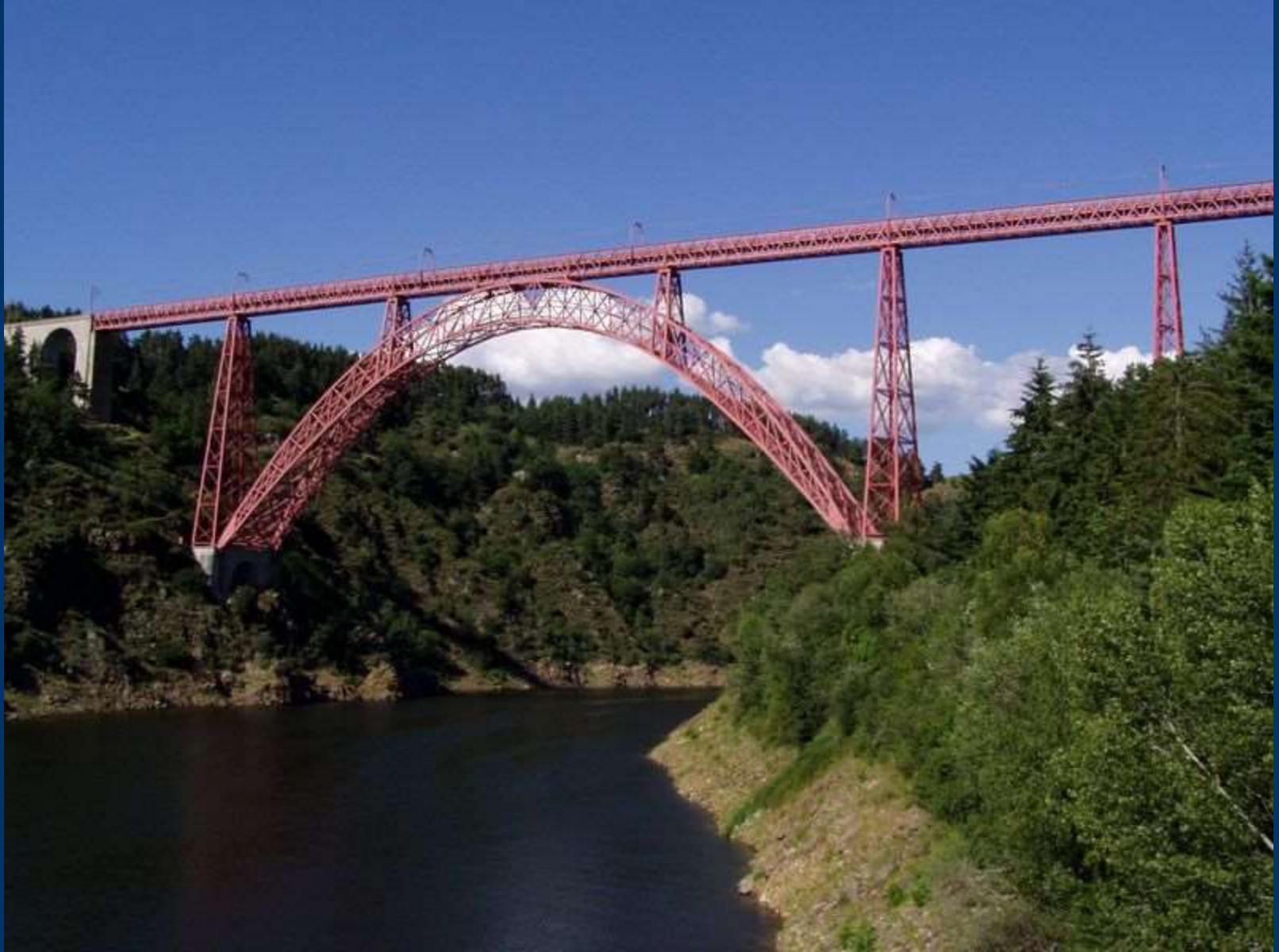
Gustave Eiffel. Garabit viaduct (a railway arch bridge). 1880- 1884 It is a railway arch bridge spanning the Truyere river.
