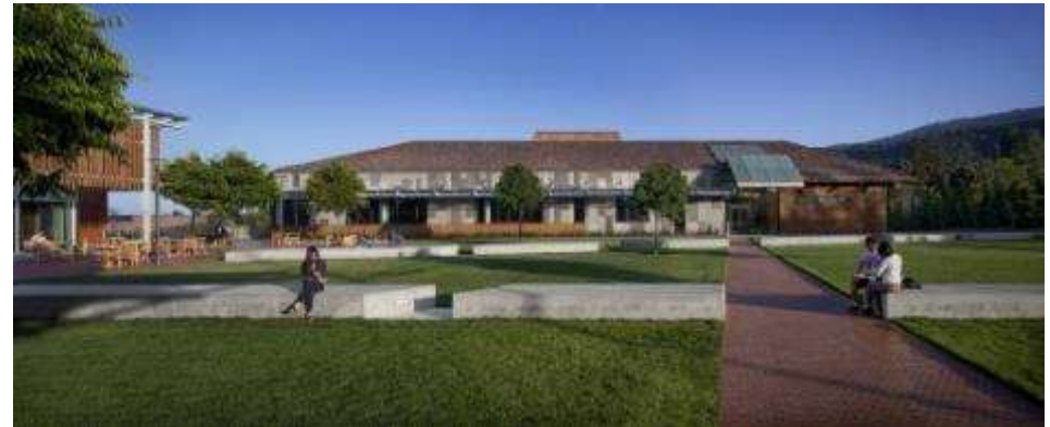
FH – Physical Sciences + Engineering Center
