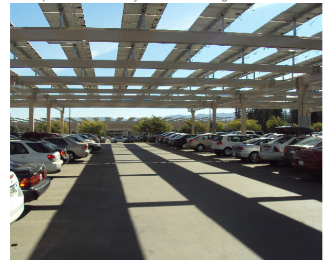
Solar photovoltaic arrays above Parking Lots A + B
