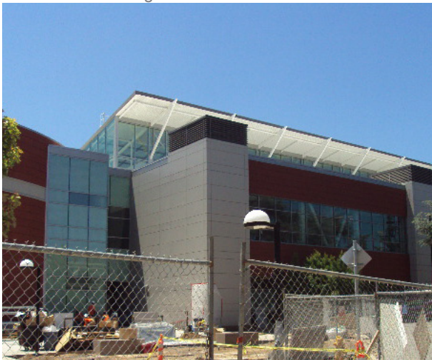
Media and Learning Center under construction
