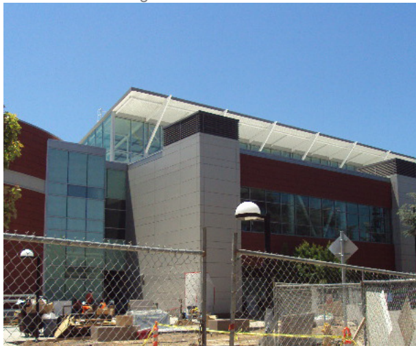
Media and Learning Center under construction
